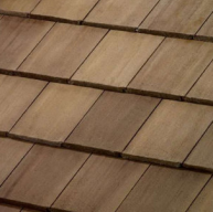
CONCRETE TILE ROOF
